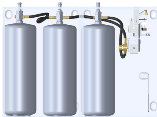
Figure 5.4: Routing of expellant gas hoses for a KitchenX triple system.
